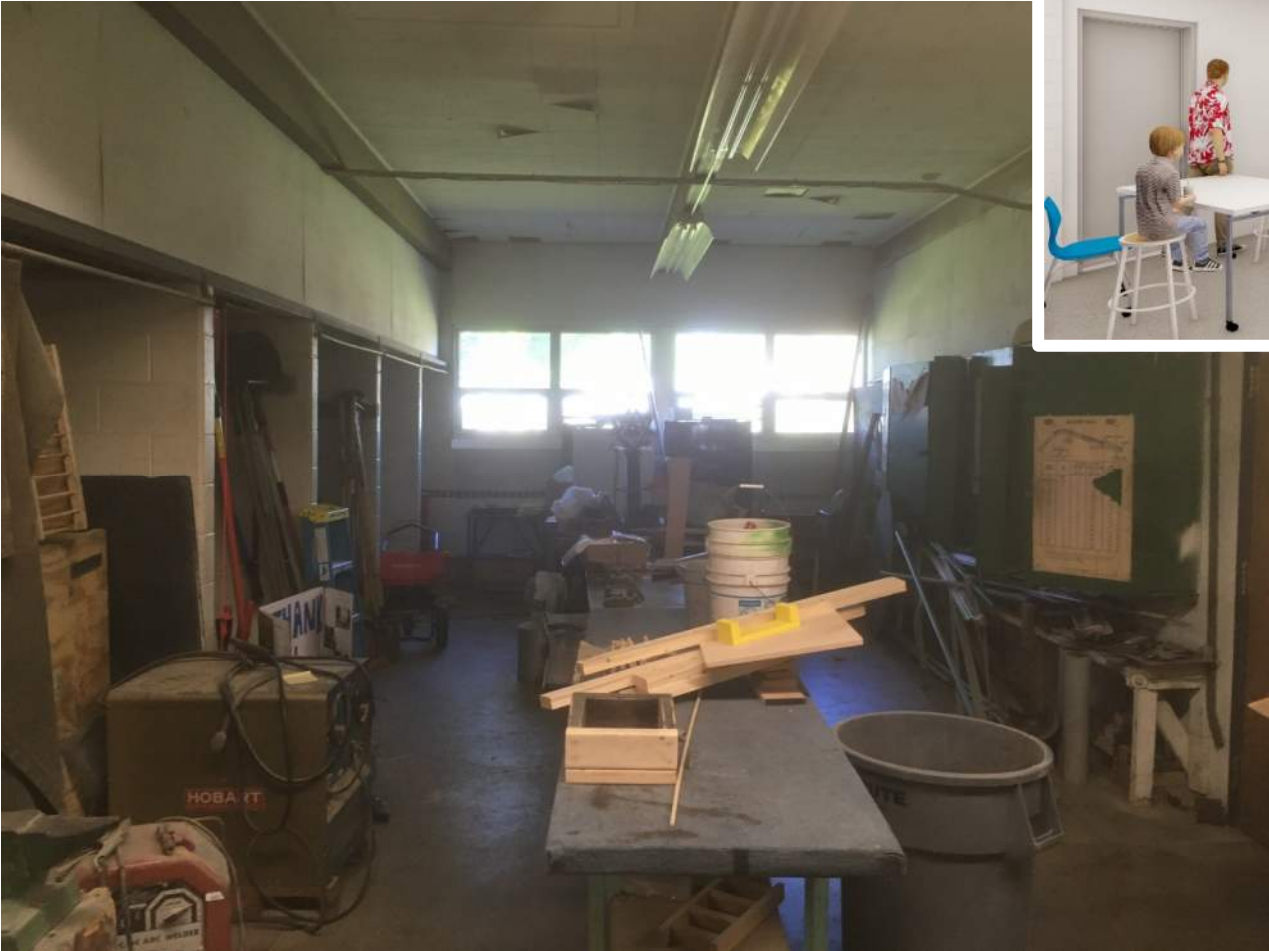
STEM Wing Renovation - Before
