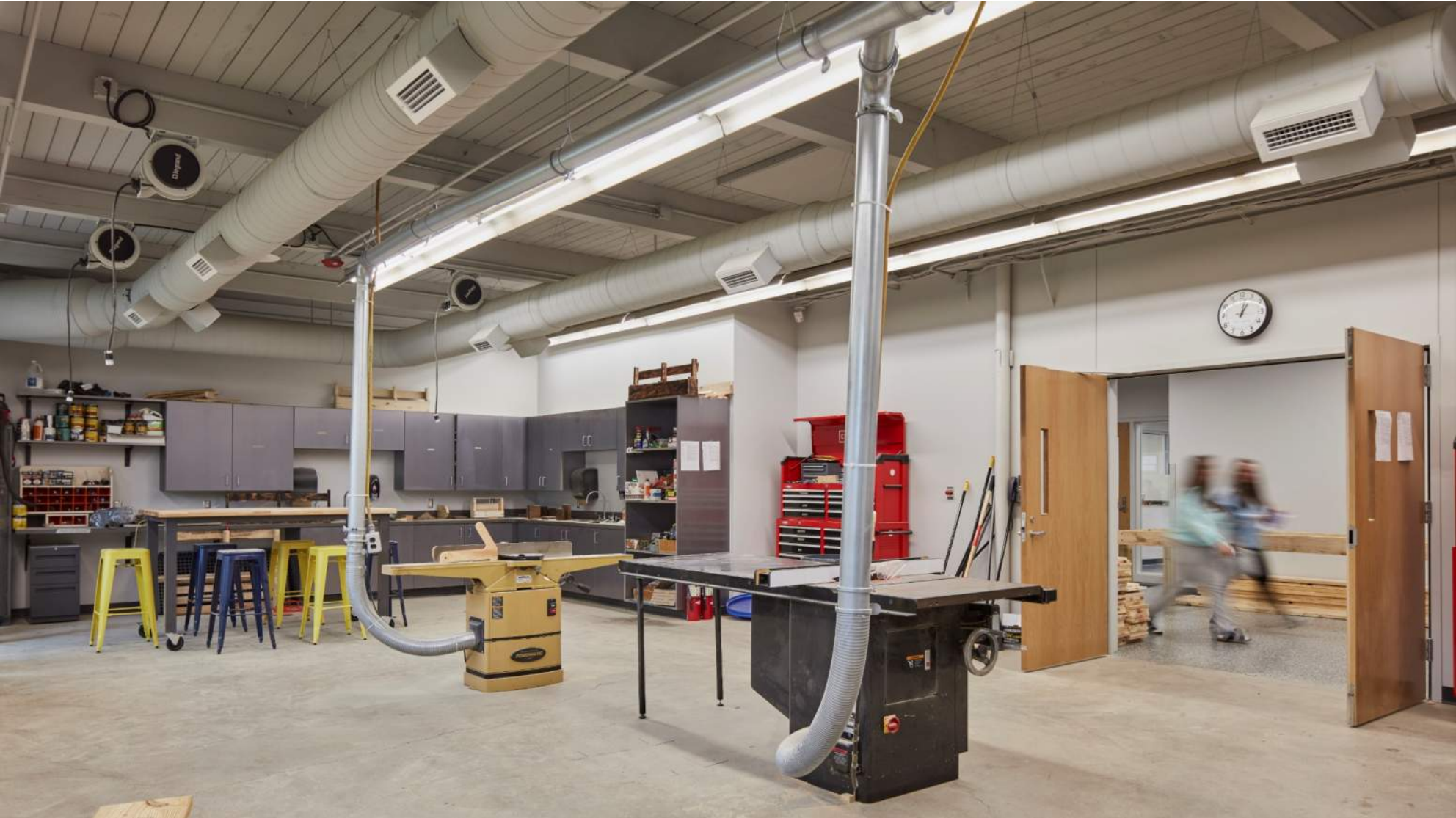
STEM Wing Renovation - After
