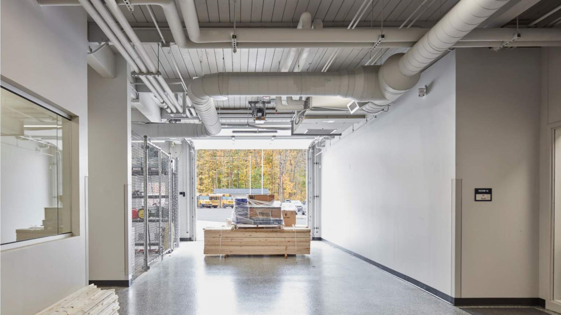
STEM Wing Renovation - After
